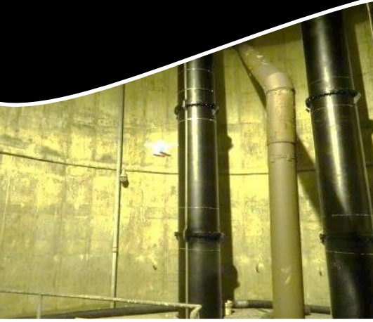
Confined Space Inspection
