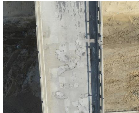
Bridge Condition Assessment
